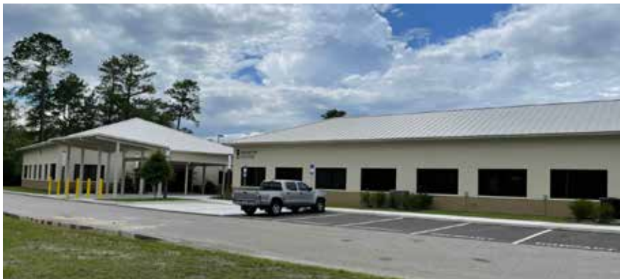
Completed Parish Office and Ministry Buildings
